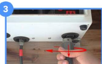
Disconnect the grey module cable at the bottom of the module, by turning the connector body counter-clockwise.
