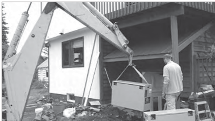
The new battery bank is installed at the Alaska Homestead Lodge to help power the lodge and the IMPROVE monitoring site.
